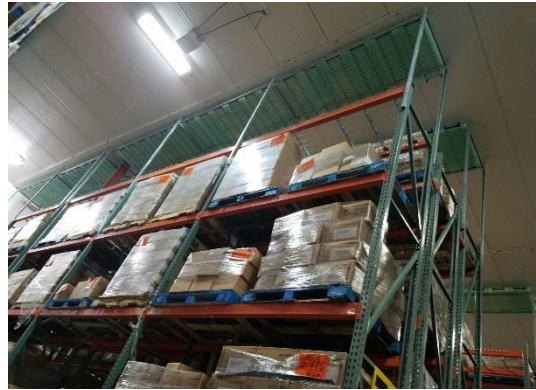
Rack extension lay-down PCM modules
