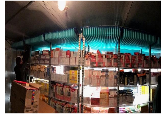
Grocery reach-in freezer
