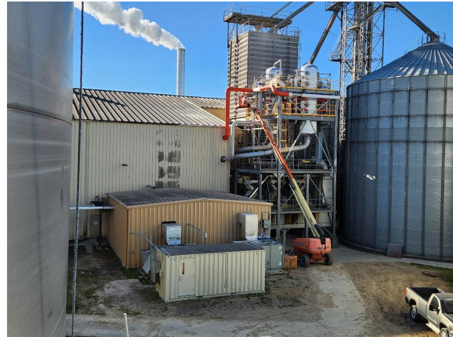
Kinergetics Slurry Heater eliminates need for high temperature steam and reduces PC.
