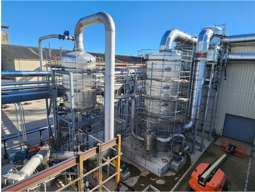
ExFactor™ heat recovery system with multi-stage MVR for process steam generation.
