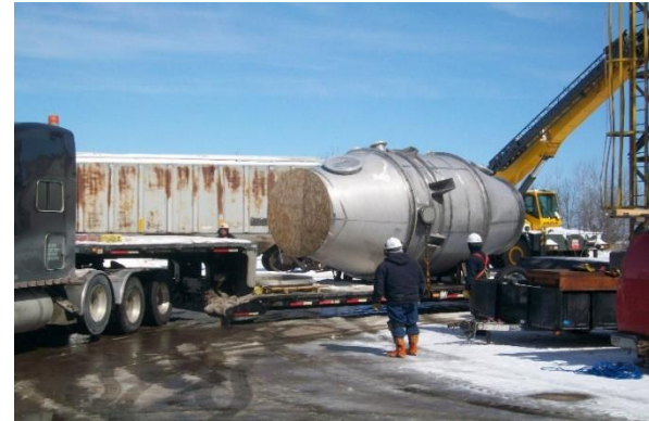
RTO Exhaust Heat Recovery
