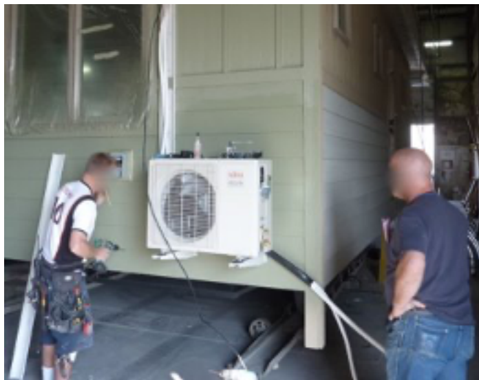
Figure 2: Example heat pump installed on a manufactured home.
