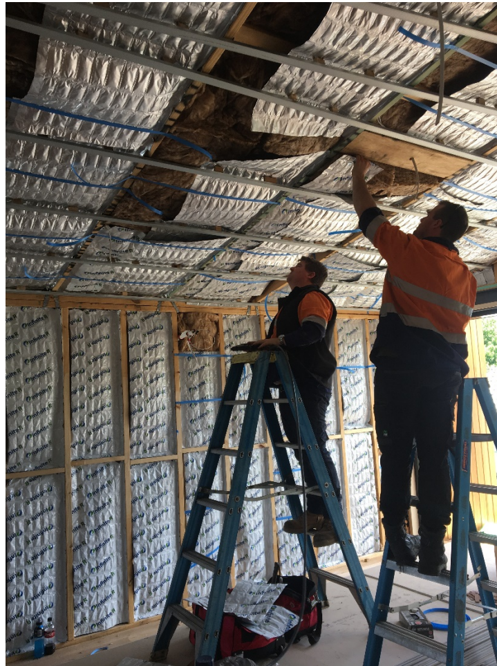
Figure 22. Installation of PCM in Ceiling and Wall Applications
