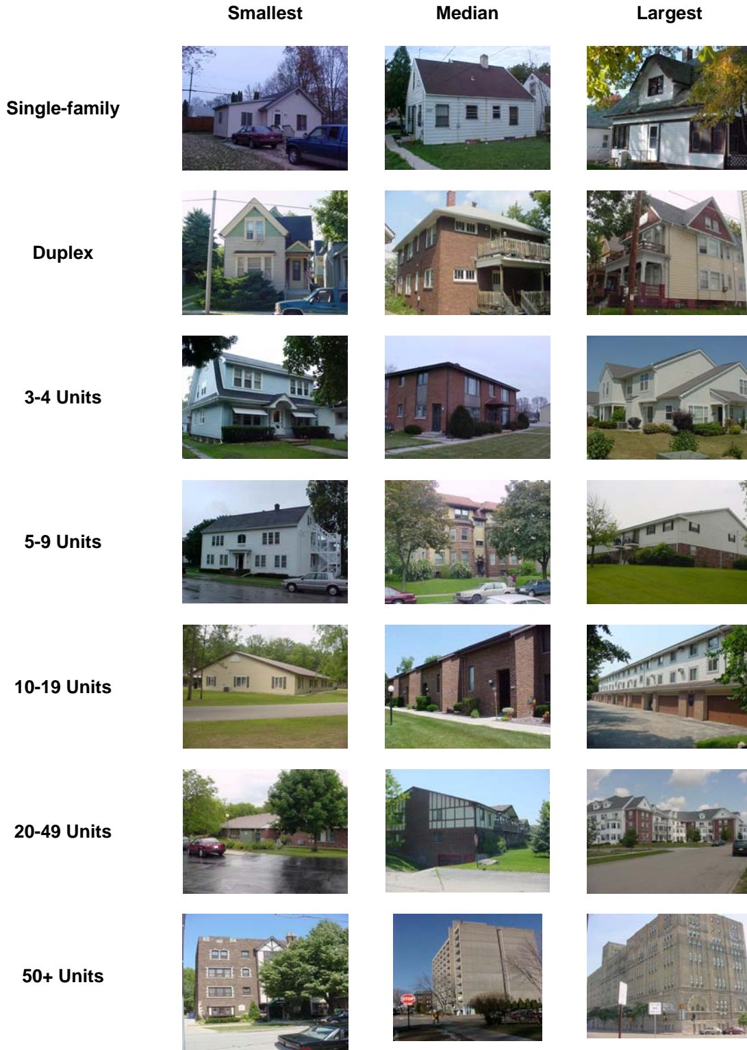
FIGURE 1. SMALLEST, LARGEST AND TYPICAL STUDY BUILDINGS BY SIZE CATEGORY
