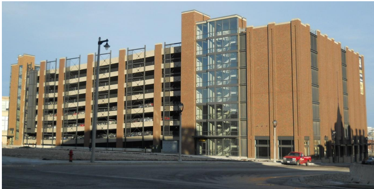
Figure 1. The Brewery parking structure
