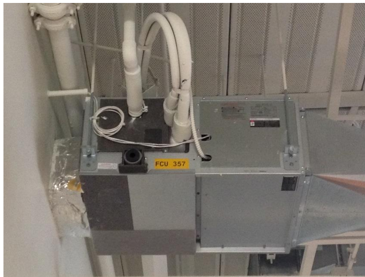
Figure 5. Typical branch selector. Note that this unit has five pairs of refrigerant lines (and one blank) and so serves five fan coil units.
