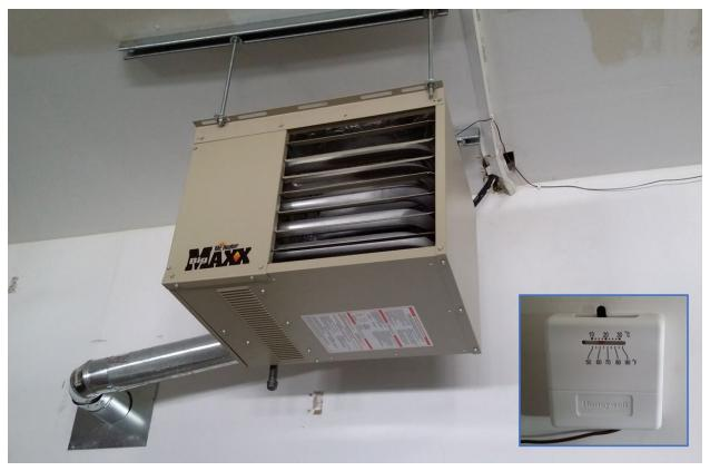
Figure 31. Example of a garage heater, with thermostat set to 60F (Site 125).
