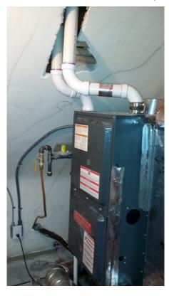
Figure 46. Furnace installed in an uninsulated walk-up attic at Site 172.
