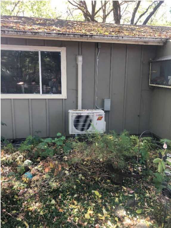
Figure 16. The outdoor unit of the mini-split system at Site 3.
