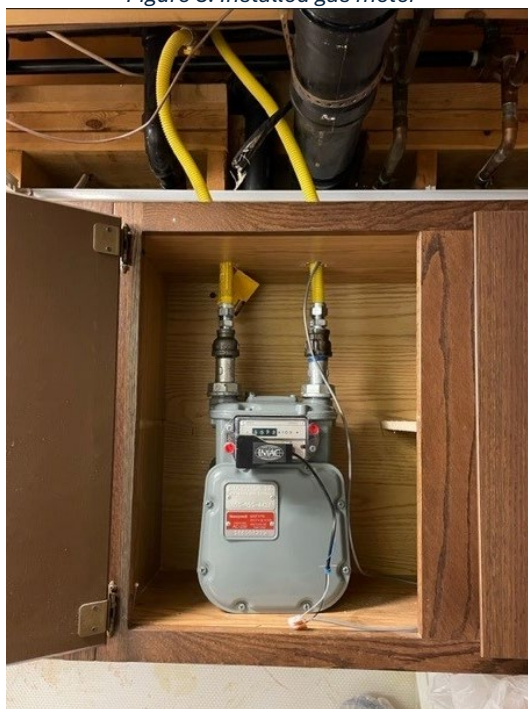
Figure 3: Installed gas meter
