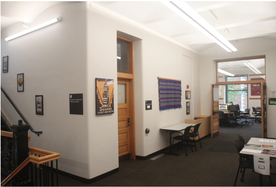
The new suspended linear lighting not only provides energy savings, but significant improvement in lighting quality with direct/indirect, task tunable fixtures.
