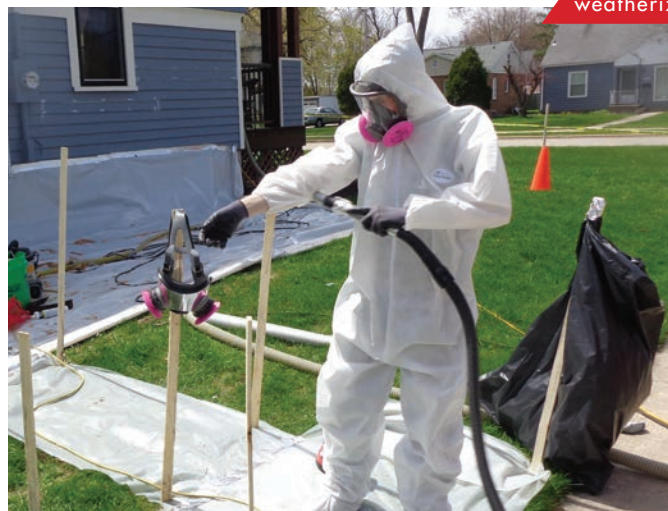
Worker using a HEPA vacuum to clean residual dust off personal protective equipment.
