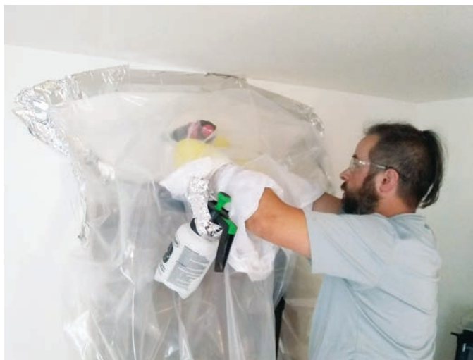
Dave Williams of ADVOCAP's weatherization department demonstrates how a glove bag can be used to control dust.
