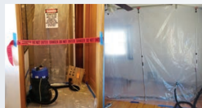
(left) A HEPA vacuum is incorporated into the containment enclosures. (right) An asbestos glove bag is used to install a bathroom exhaust fan.
