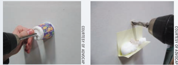
(left) You can use a small cup as a shroud filled with shaving cream! (right) Here is a Post-it Note with a bead of shaving cream that catches debris.
