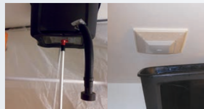
A storage tote being used as a shroud during a bathroom fan upgrade.
