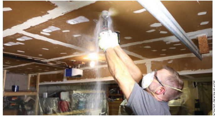
Drilling without a shroud.
