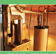
For the greatest energy savings, choose a high-efficiency furnace with a 95 percent or greater annual fuel utilization efficiency (AFUE) and an electronically commutated blower motor (ECM). When properly installed, furnaces with an ECM:
