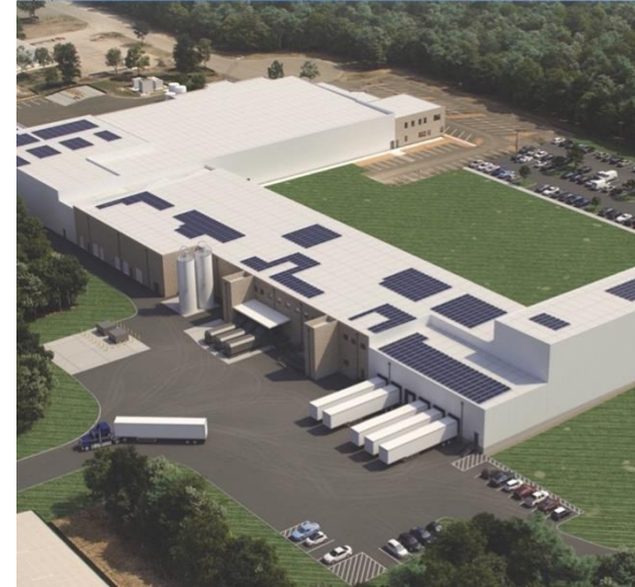
50 TALBOT LANE, S. WINDSOR, CT 190,000 SQUARE FEET
