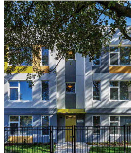
Exterior of Tierra Linda, the first PHIUS+ certified multi-family building in Chicago Image credit: Landon Bone Baker Architects
