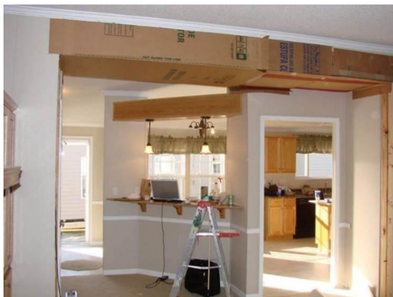
Figure 16. Interior duct chase mock up by Southern Energy Homes (Moyer, et al. 2008)
