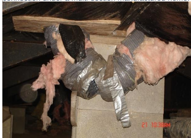
Figure 8. Example of a failed cross-over duct connection under a multi-section manufactured home.
