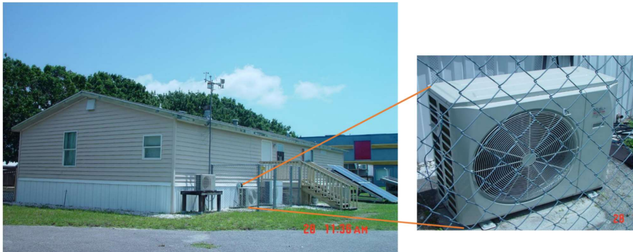
Figure 28. Picture of FSEC MH lab and the heat pump's outdoor unit
