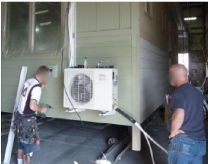
Figure 2: Example heat pump installed on a manufactured home. Photo courtesy of Brady Peeks, Northwest Energy Works
