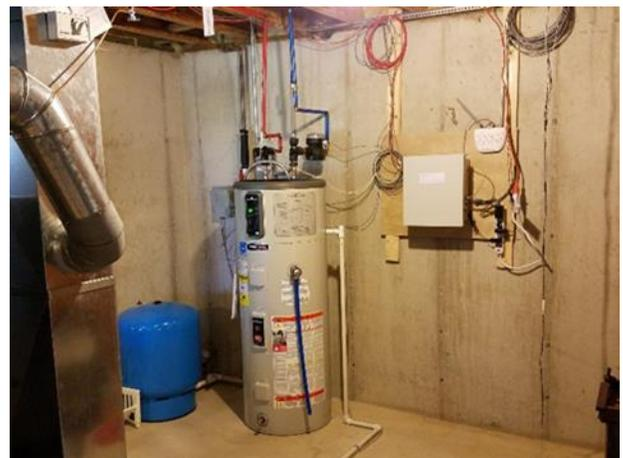
Figure 4. Water heater and monitoring components.
